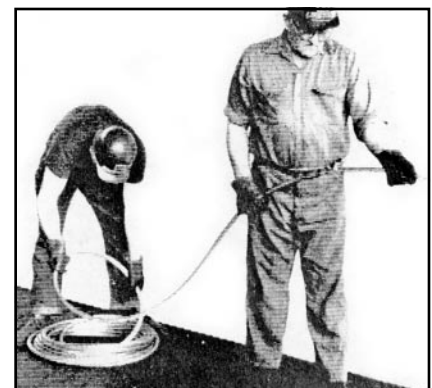
Illustrating a wrong method of uncoiling rope.
